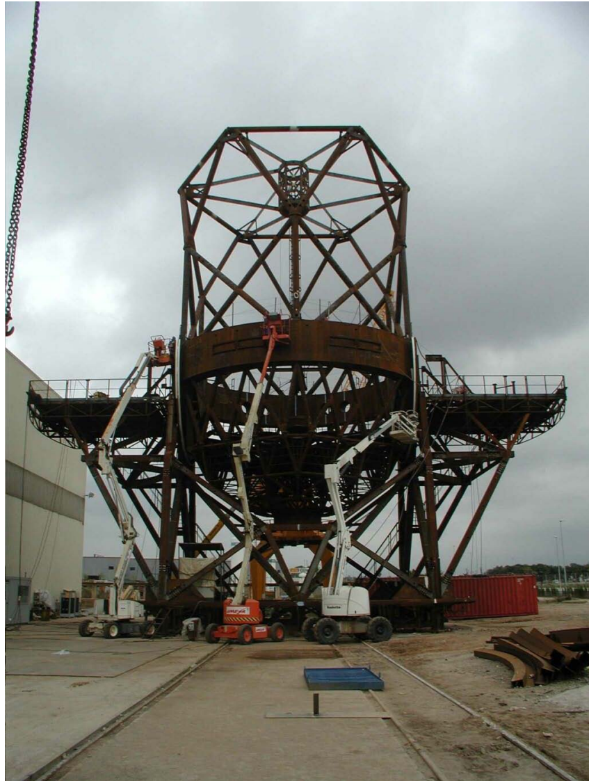
Fig. 4. Picture of the telescope structure being mounted at the factory in Tarragona. The picture date is 2002 September 1.
