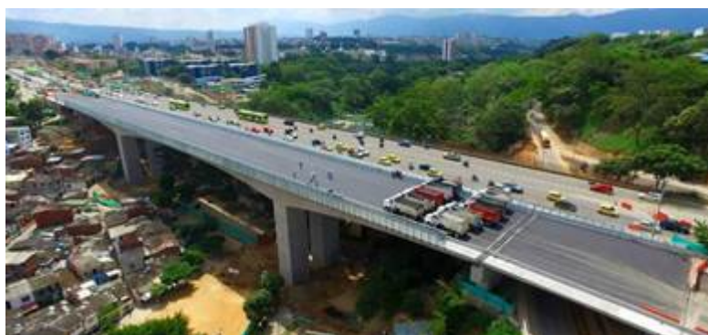
Figure 1 La Unión Viaduct (Left Side). Authors.
