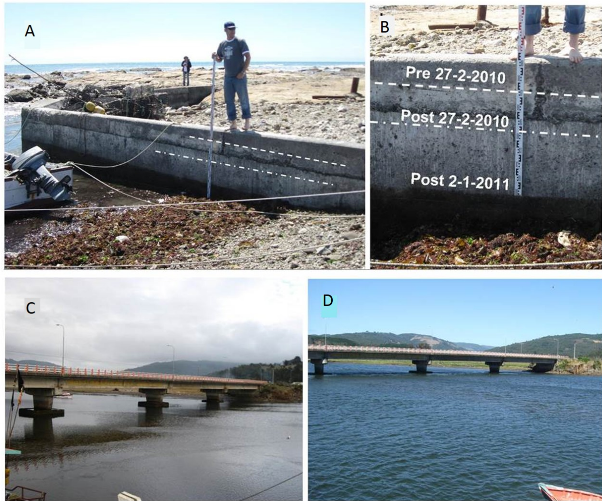
Fig. 9. Evidences of vertical changes at Mocha Island and Tirúa after Araucanía 2011 earthquake. A-B. Same place at Mocha Island shown in figure 7D. It is clear the sea level drop of 50 cm. C-D. Tirúa bridge. Left photo taken on April 27th 2010 one hour after the low tide. Right photo: same view on January 20th 2011 at the time of low tide. Note the upper position of the water in the columns evidenced 20 cm of subsidence after the M_w=7.1 event. The Tirúa River had more caudal on January 2011, even if we consider that this is the summer dry season.
