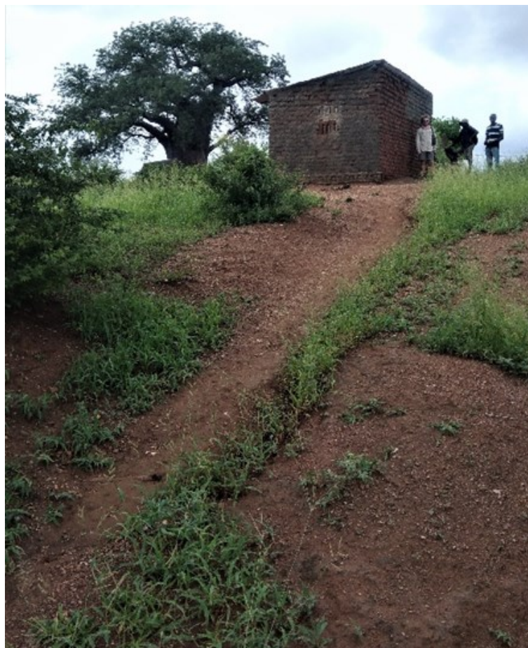
Figure 14 – House settled in a high erosion-risk area. Source: Personal Archive of Júlia Paiva, February 2018.
