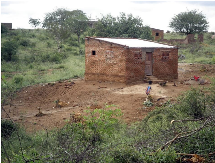
Figure 6 – House built in bricks in Moatize rural area and landslide after rainstorm. Source: Personal Archive of Clara Medina, February 2018.
