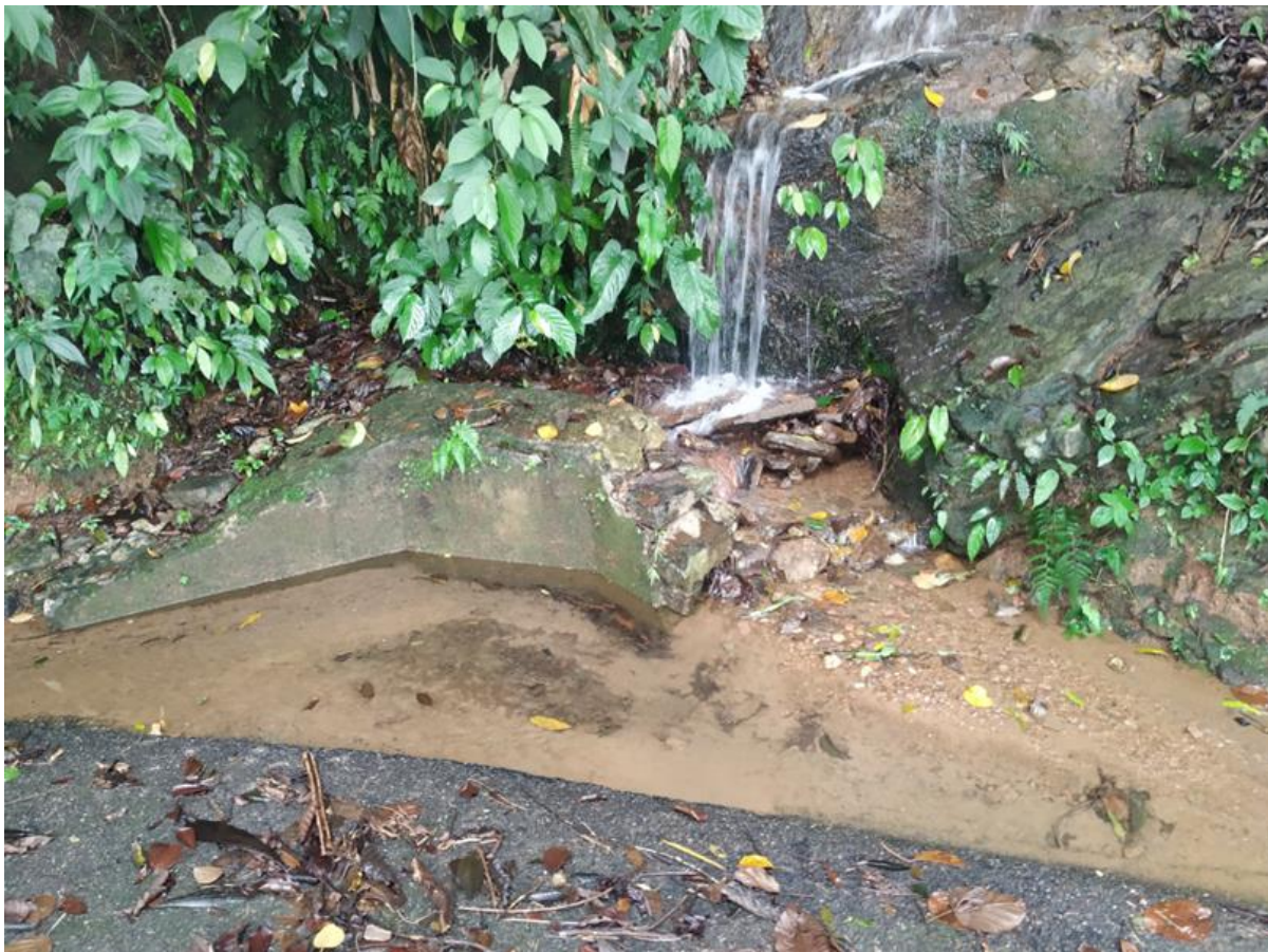
Figure 6 – Manhole completely clogged by sediments coming from a drainage in Central sector. Source: Authors (2022).
