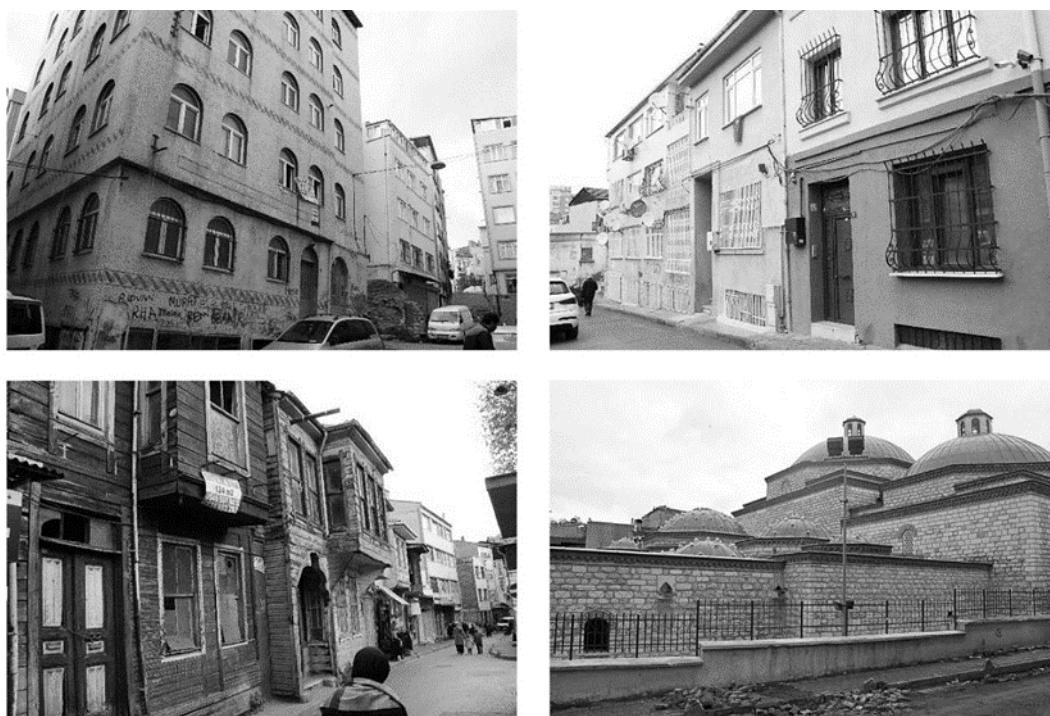
Figure 12 – Buildings materials: concrete (top left), masonry (top right), timber (bottom left), and stone (top right). Source: Authors (2023).
