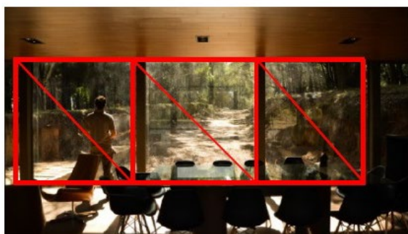
Figure 25: Comparative structures. With diagonals (Pratt), without them (Vierendeel). Pabellón. (Source: Ferrer & Alarcia, 2014)
