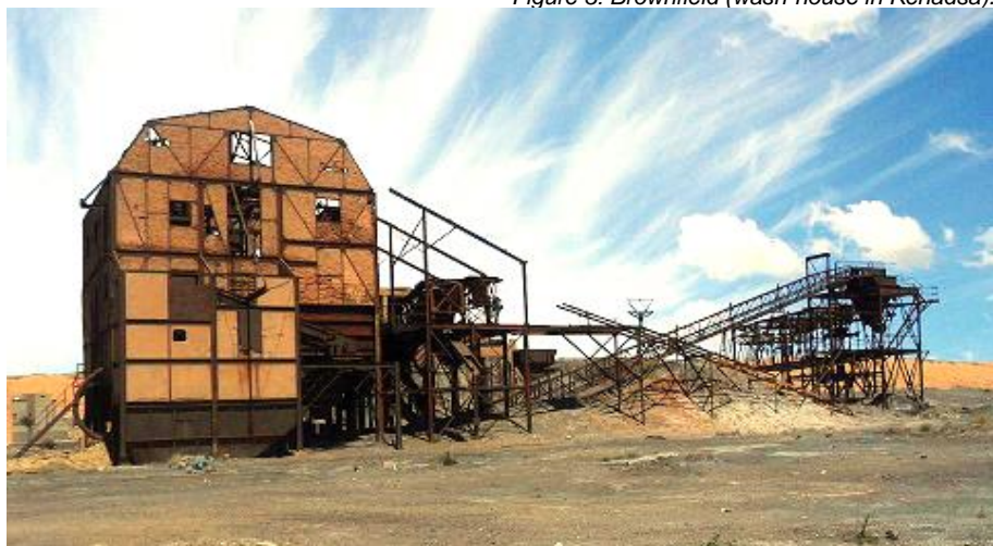
Figure 3: Brownfield (wash-house in Kenadsa).
