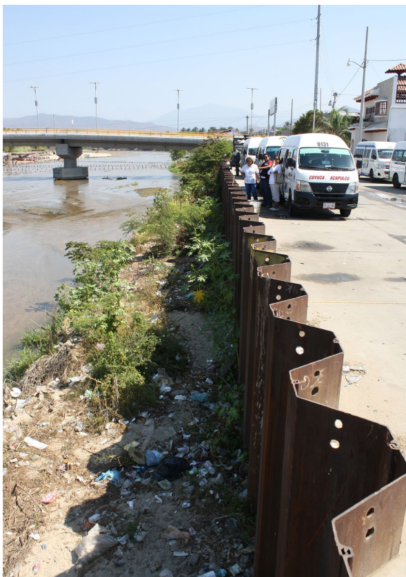
Figure 3. Protection curtain and Coyuca I Bridge in April 2017. Source: Photograph courtesy of the Coyuca Climate Resilient Project.
