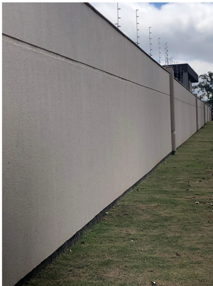
FIGURE 04 Dourados-MS: Ecoville Residence gated community wall. The author (2020)
