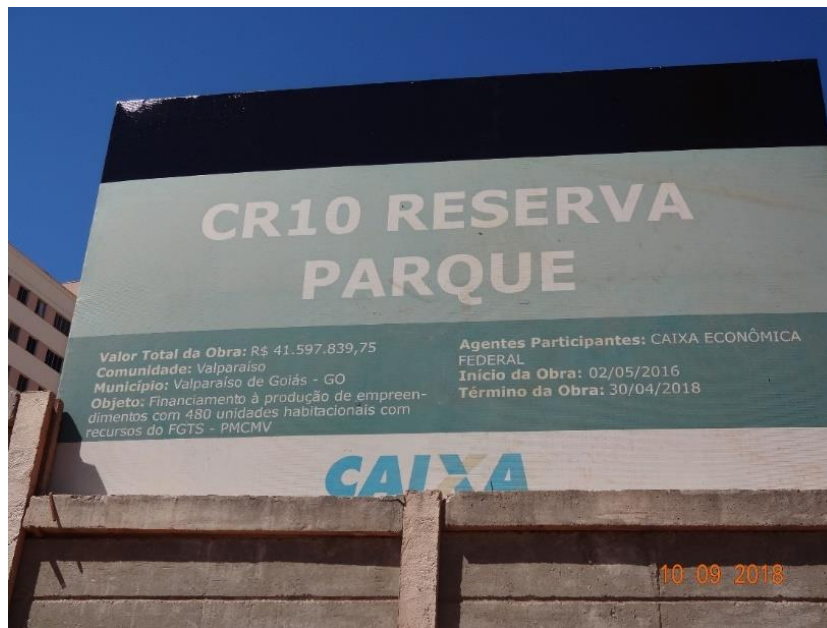
Figure 5. Identification plate of the vertical development site in Valparaíso de Goiás – 2018.
