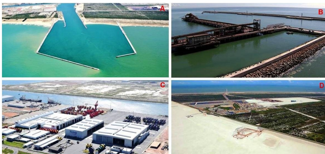
Figure 2 – The Açú Port facilities: A (terminals TX1 and TX2), B (breakwater at TX2), C (companies installed along the navigation channel), D (hydraulic landfill built near the restinga area).
