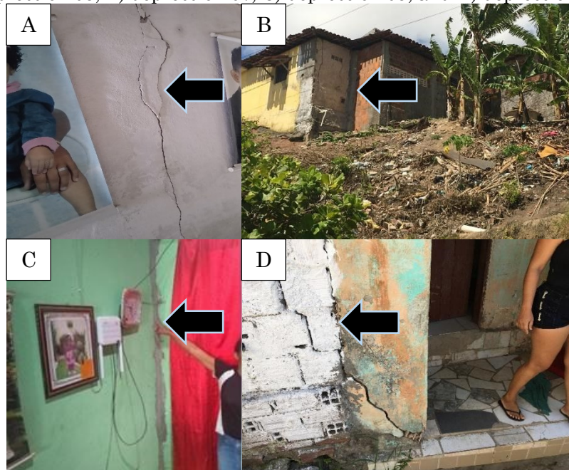
Figure 07 – Cracks identified in the buildings were indicated by the arrows on the images. A) depression 05, B) depression 07, C) depression 09, and D) depression 12.
