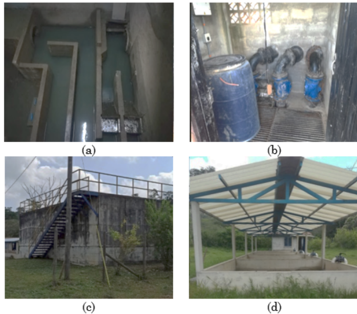
FIGURE 4. Treatment units in San Roque municipality WWTP. a) Preliminary treatment. b) Pumping station. c) UASB reactor. d) Drying beds
