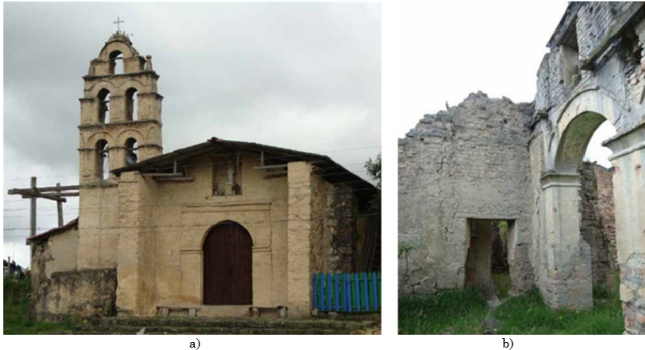
Figure 1 Doctrinal chapel in Tausa: a) frontal sector; b) rear sector Source: Created by the authors.
