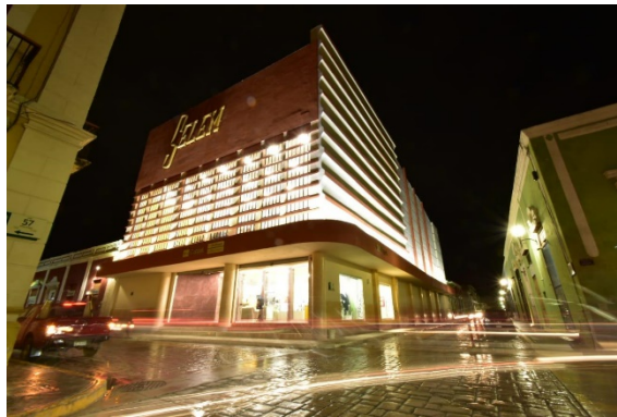
FIGURE 7 View of the intervention building
