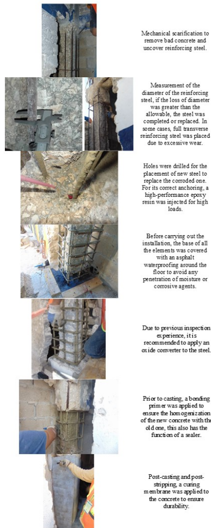
FIGURE 6 Uniform deep repair process
