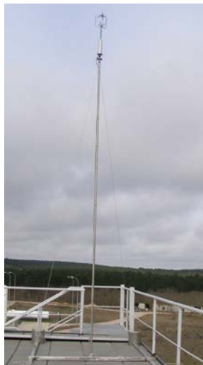
Figure 6 Meteorological mast for Enair EPRO70 Wind Turbine
