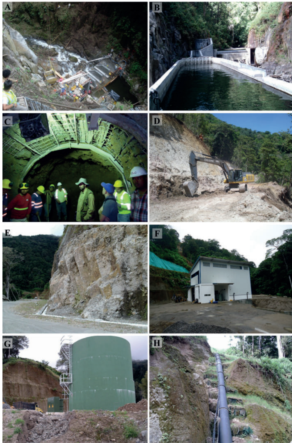
Fig. 8: A. Dam construction and finished works (B), Tunnel construction process (C-D). Pipeline slope excavation process (D-E). Final finishing of slopes in columnar agglomerate (E). Surge tank (G) and penstock (H).
