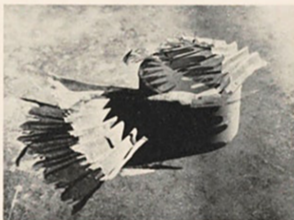
FIG. 22. The telltale regularity of a cylindrical object may be camouflaged with paint, with partial obliteration, with false shadow formation, or with all three, as was done here. The paint distorts the object through optical illusion, while the scaffolding at the top and side, covered with canvas or some other garish, partially conceals the object and likewise throws confusing shadows
