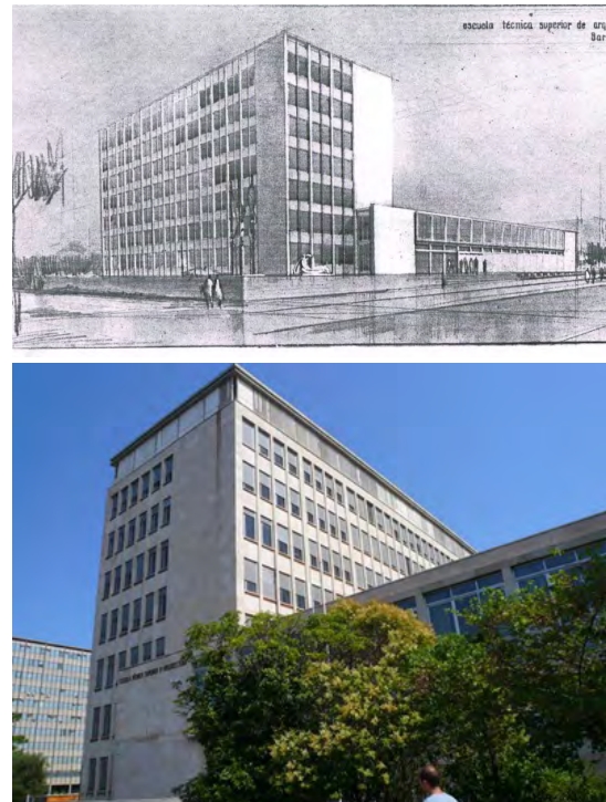
Fig. 8 Building during the design phase and at present time (right) [19].
