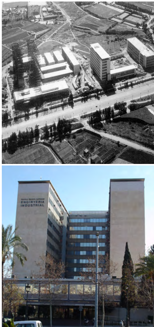
Fig. 5 Photo of the building during the construction (left) and at present time (right). Fuente: Barcelona Superior Technical College of Industrial Engineers.
