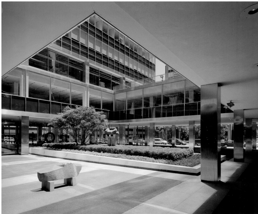
Figura 3 Lever House, Skidmore, Owings & Merrill, New York, NY 1952. Fotografía Erza Stoller
