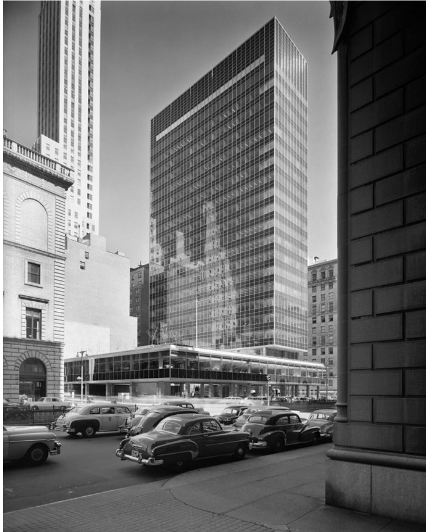
Figura 1. Lever House, Skidmore, Owings & Merrill, New York, NY 1952. Fotografía Erza Stoller
