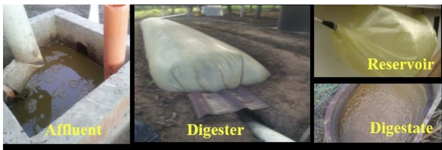
Figure 1. Tubular digester setup located on "Marcella" farm.
