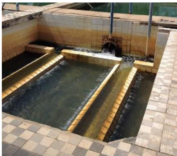
Figure 1. Image of one of the filters during the backwash process.
