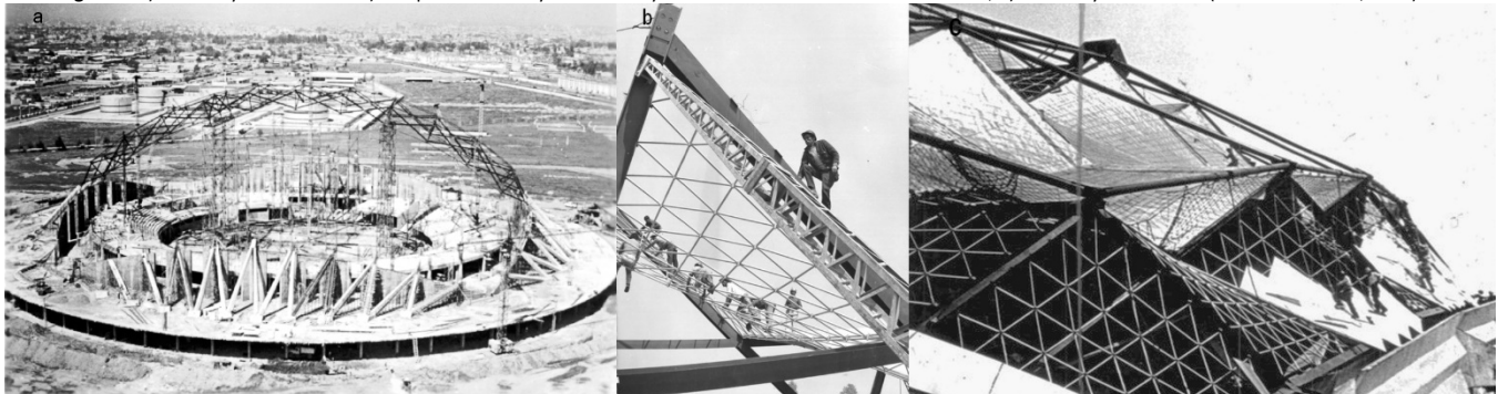
Figure 7. a) Assembly of the arches b) Sample of assembly of secondary structures over the structure of arches; b) Assembly of the deck. (Villasana Suverza, 2015).
