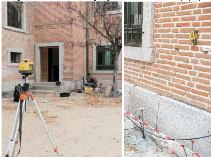
Figure 9. Control of structural lifting using a laser level. Source: Author's property.
