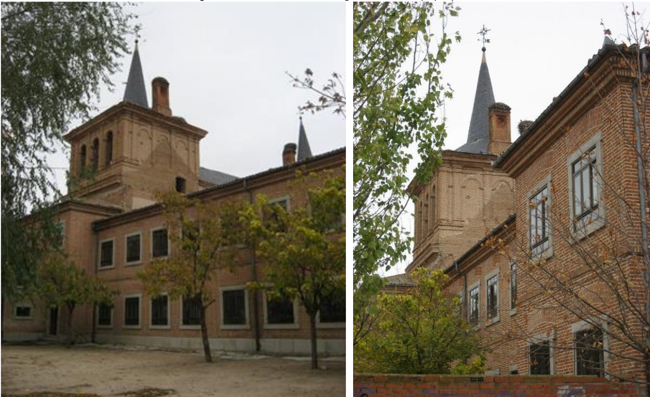
Figure 6. Panoramic view of the building. Source: Author's property.
