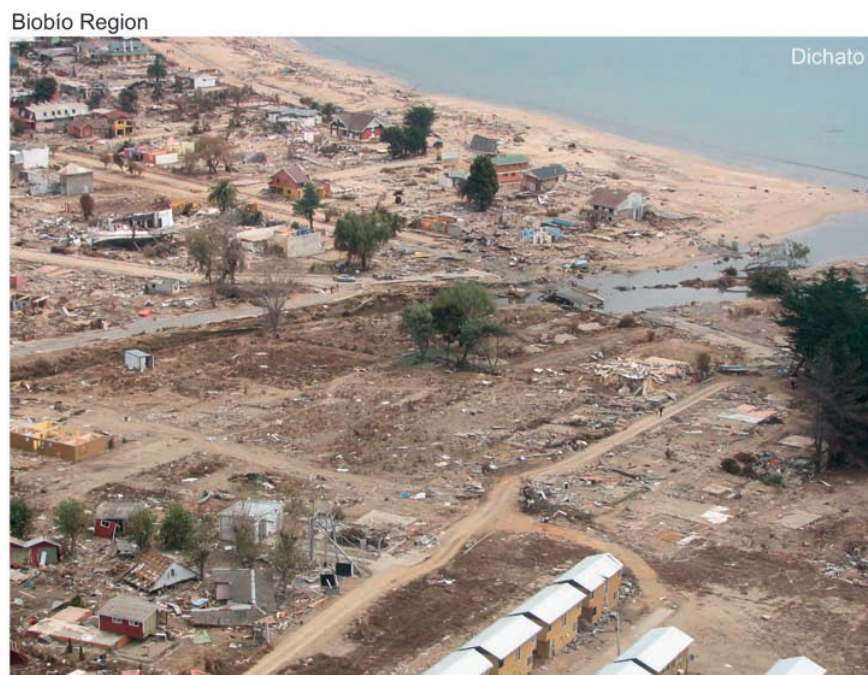
FIG. 10. Photograph showing dramatic tsunami impact at Dichato, along the coast of the Biobío Region.
