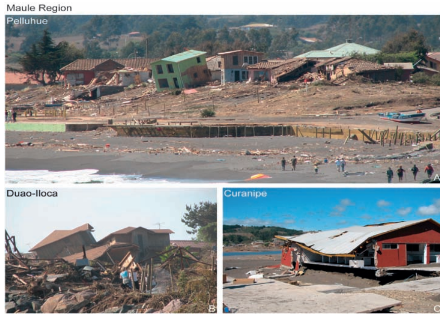
FIG. 9. Photographs evidencing strong tsunami impact along the coast of Maule Region. A. , B. Littoral area affected by tsunami inundation at Pelluhue and Daao-Iloca, respectively; C. Tsunami impact at Curanipe, evidencing a strong effect of erosion processes on foundations of coastal infrastructure.
