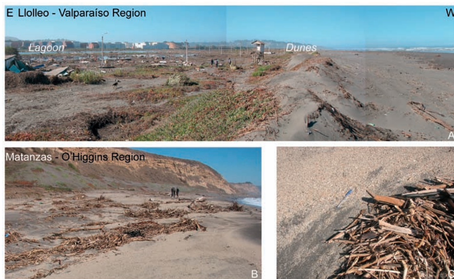
FIG. 12. A. Strong tsunami impact on dwellings at Lolloe, in Valparaiso region. In this area we observed centimeters thick sandy deposits resulted from the run-up of the tsunami overlying organic and fine sediments along the margin of the lagoon. B., C. Sandy and organic rests disposed by tsunami waves on the supralittoral zone along the coast of Matanzas.
