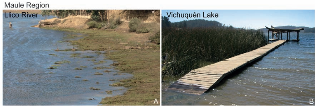
FIG. 6. A. Land subsidence evidenced by flooded fluvial terraces at the Llico River, and B. by partially submerged piers along the margin of the Vichuquén Lake, close to the coast.
