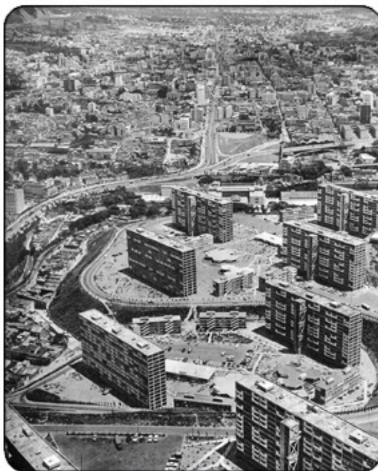
Figure 2 - The Super Bloque of January 23 shortly after construction
