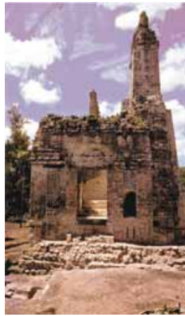
FIGURE 7. South side of Structure 6N-1 following consolidation in 1976
