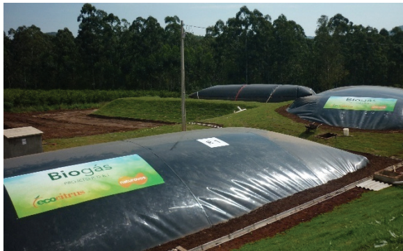
Figure 1. The reactors: on the left is the plug flow reactor R1 (PFR) with 450 m 3 ; and on the right is the vertical upflow reactor R2 (VUR) with 900 m 3 .
