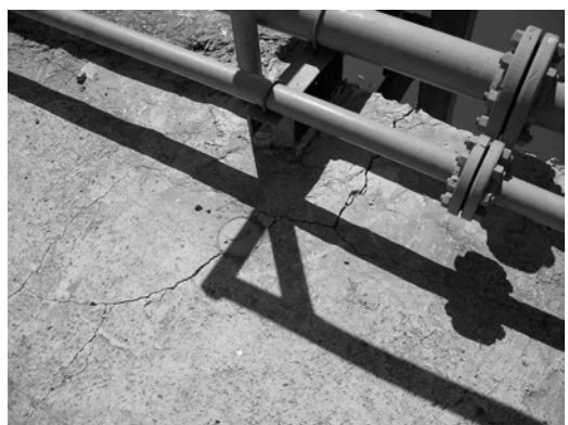
Figura 6. Losa 16 fisura diagonal
