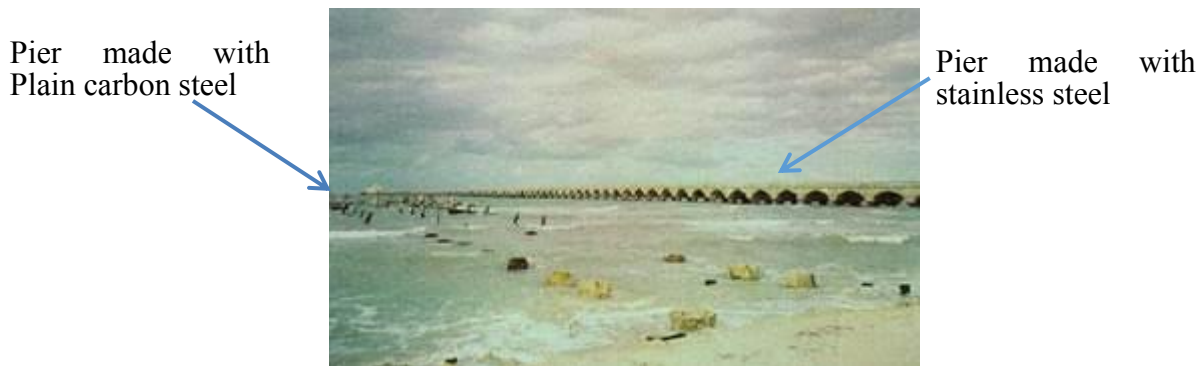
Figure1. Comparison between the pier with structures made with stainless steel (right) and the pier with structures made with carbon steel (left) (Klueh, R. L., & King, J. F. 1982).
