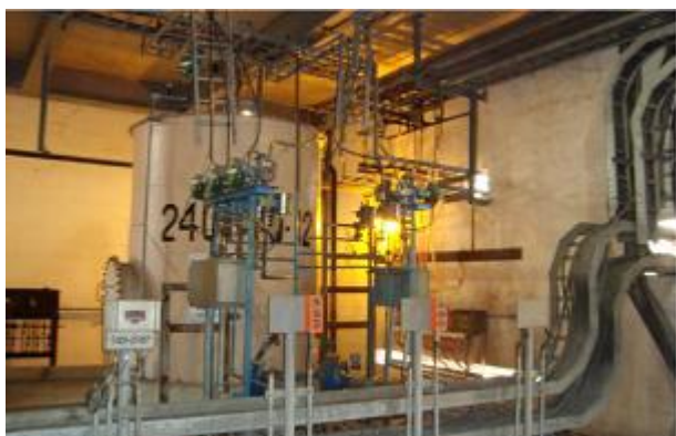
Figure 3: Dosing system with centrifugal pumps
