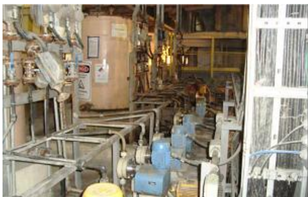
Figure 1: Dosing system with diaphragm pumps
