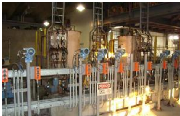
Figure 2: individual flowmeters in each line of the dosing system with diaphragm pumps
