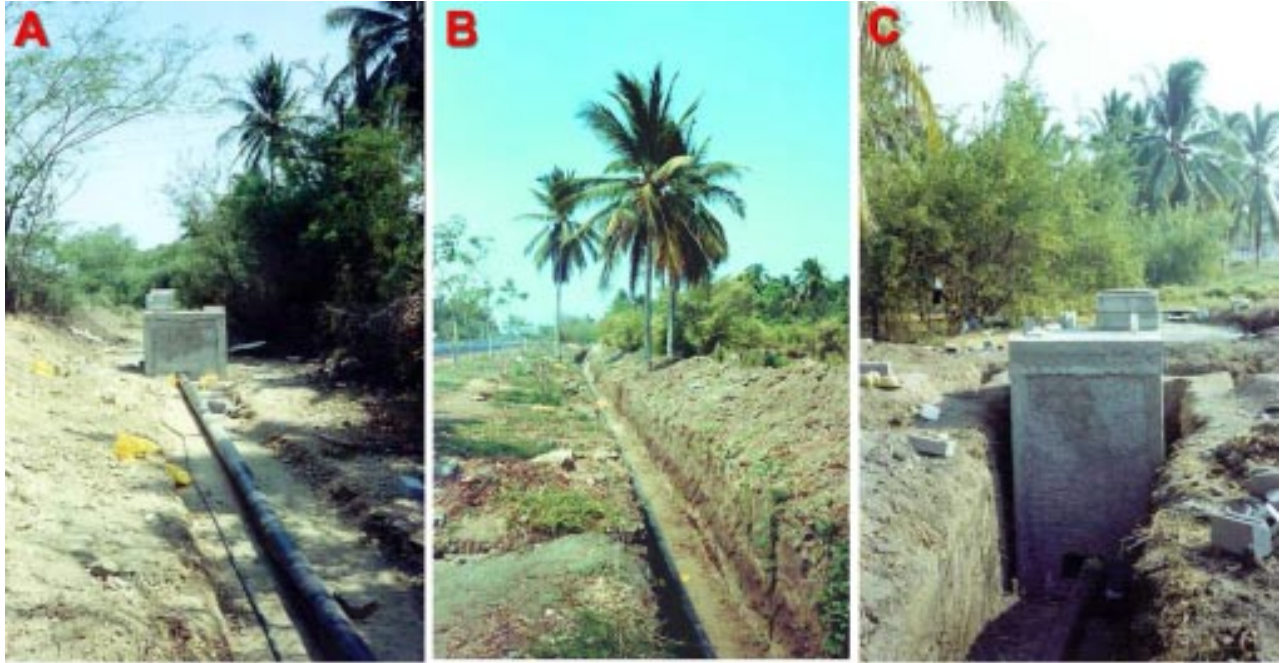
Fig. 9. Installation of the LBT. A – Polyethylene Ø8” pipe and the southern vault. B – Trench near the midpoint. The trench was accurately excavated and its bottom flattened using leveling control before pipe installation. C – Northern vault.
