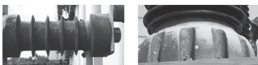
Figure 2. Insulators contaminated with algae. Rurópolis, Brazil. Source: (De Mello et al., 2008)
