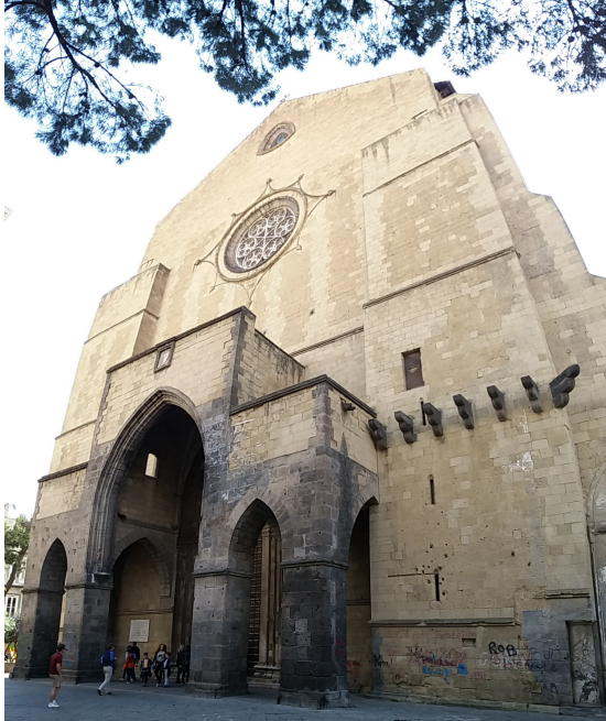
Figure 1. Reconstruction of the church of Santa Clara, Naples. Intervention by contrast. Photography by L. C. Cruz Ramírez, 2017.
