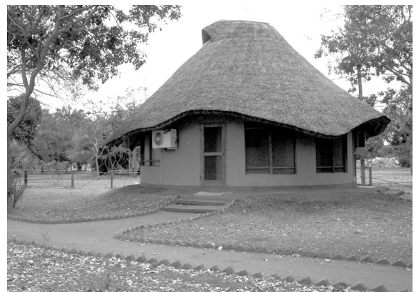
Fig. 2. A cabana at Gorongosa National Park, Mozambique. Walls are thick concrete the roof is true thatch and is also the ceiling. Note that the peak is built to allow the hot moist air to escape.
