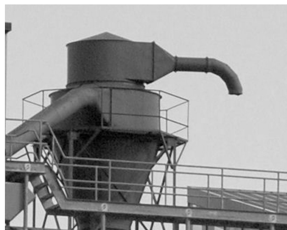
Fig. 3. A cyclone separator atop Washburn/General Mills, Mill A/Mill City Museum. The unit removed dust from the mill ventilating system. An important protection from explosions.
